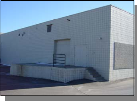
Rear Loading Docks
